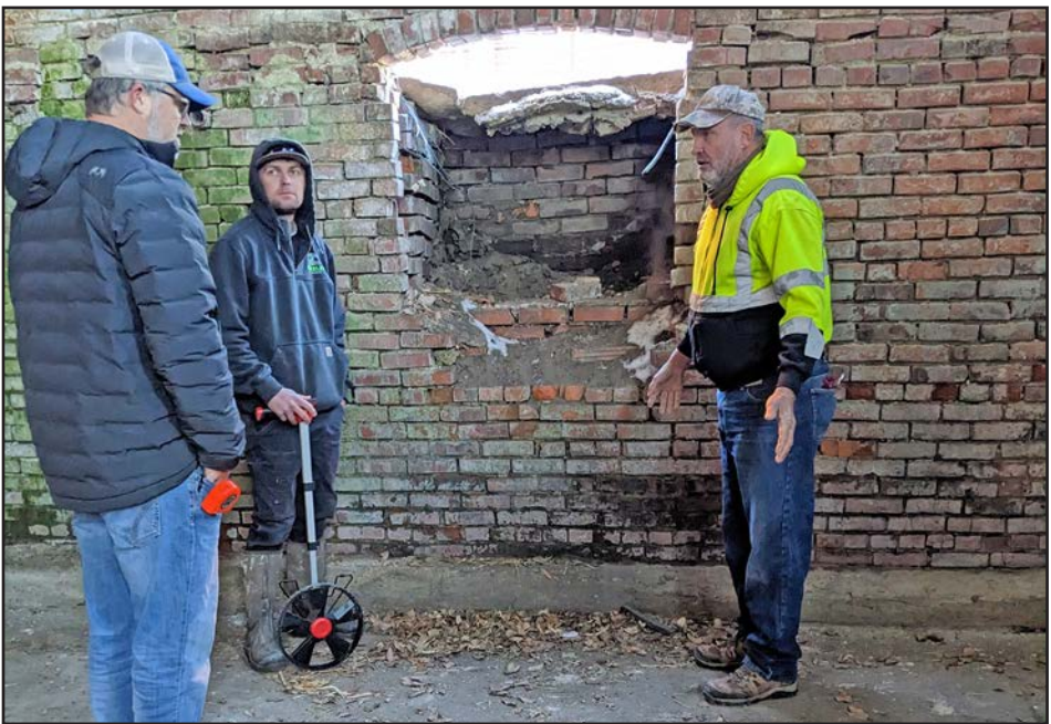
Justin Strasburg (left) discusses the removal of interior brick walls at the basement level of the Archie's building with a masonry contractor. Decisions were also made about where footers would be placed and how block walls will take their place.
