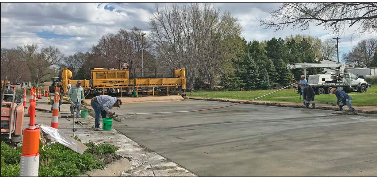
Workers screed cement after a Gomaco cement paver pour on Tuesday, April 30, east of Mills Hardware. The street project is replacing asphalt, which was breaking down due to water flow coming from the north. - Janet Larreau photo
