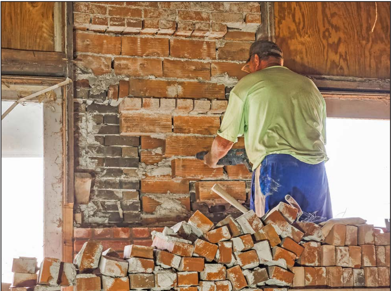
Standing on scaffolding on the north side of the old Archie's Cafe building, a skilled mason chisels out mortar between the old bricks. By the time he is finished with the restoration of the walls and entry, he will have touched every brick in the future home of the Arnold Area Historical Museum. - Debbie Connelly photo
