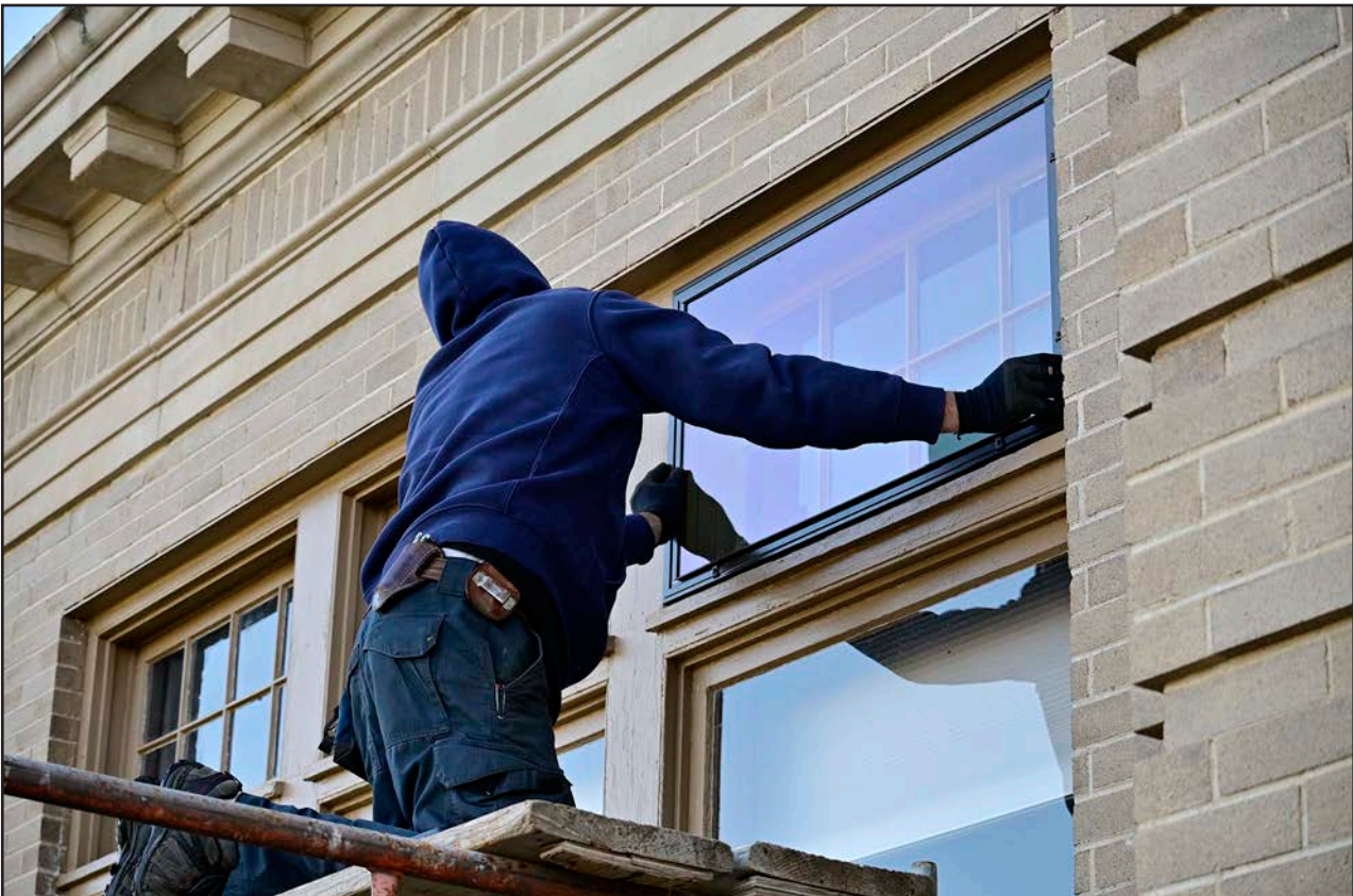
A contractor installs a new storm window over Finch Memorial Library’s original transom window. Once completed, the project will result in replacing all the building’s storm windows that date back to the 60s or 70s. - Jessica Tickle photo
