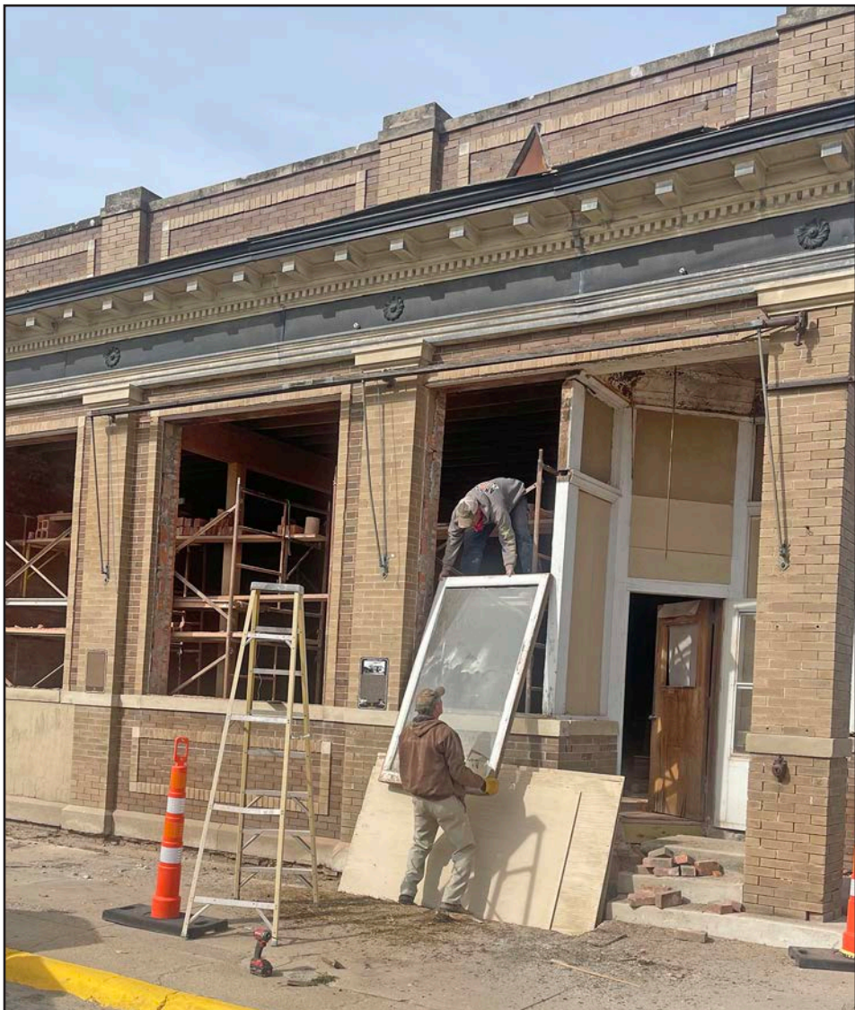
Lane Chesley hands down a heavy window to Rick Peterson last week, in preparation for brick to be repaired around all window openings at the future site of the Arnold Area Historical Museum (AAHM). Once the openings are repaired, they will be boarded back up as renovation on the old Archie's Café building continues. Both Peterson and Chesley are AAHM board members. - Becky Dailey photo
