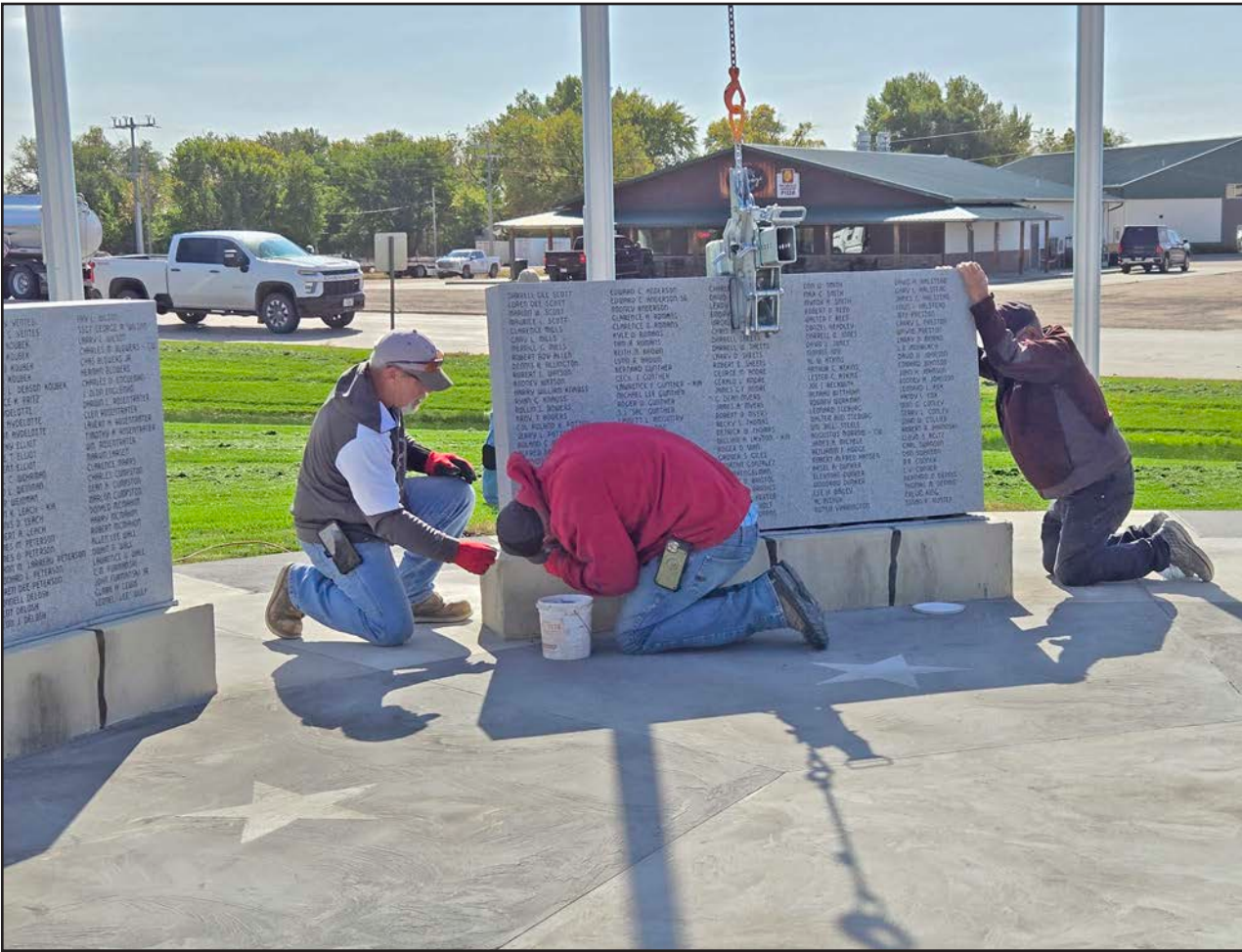
Palmer Monument workers Shane Kelly and Trent Keezer, with help from Mike Harvey, set a monument in place. Also pictured are decorative concrete stars that have been applied in front of each wall of names.
