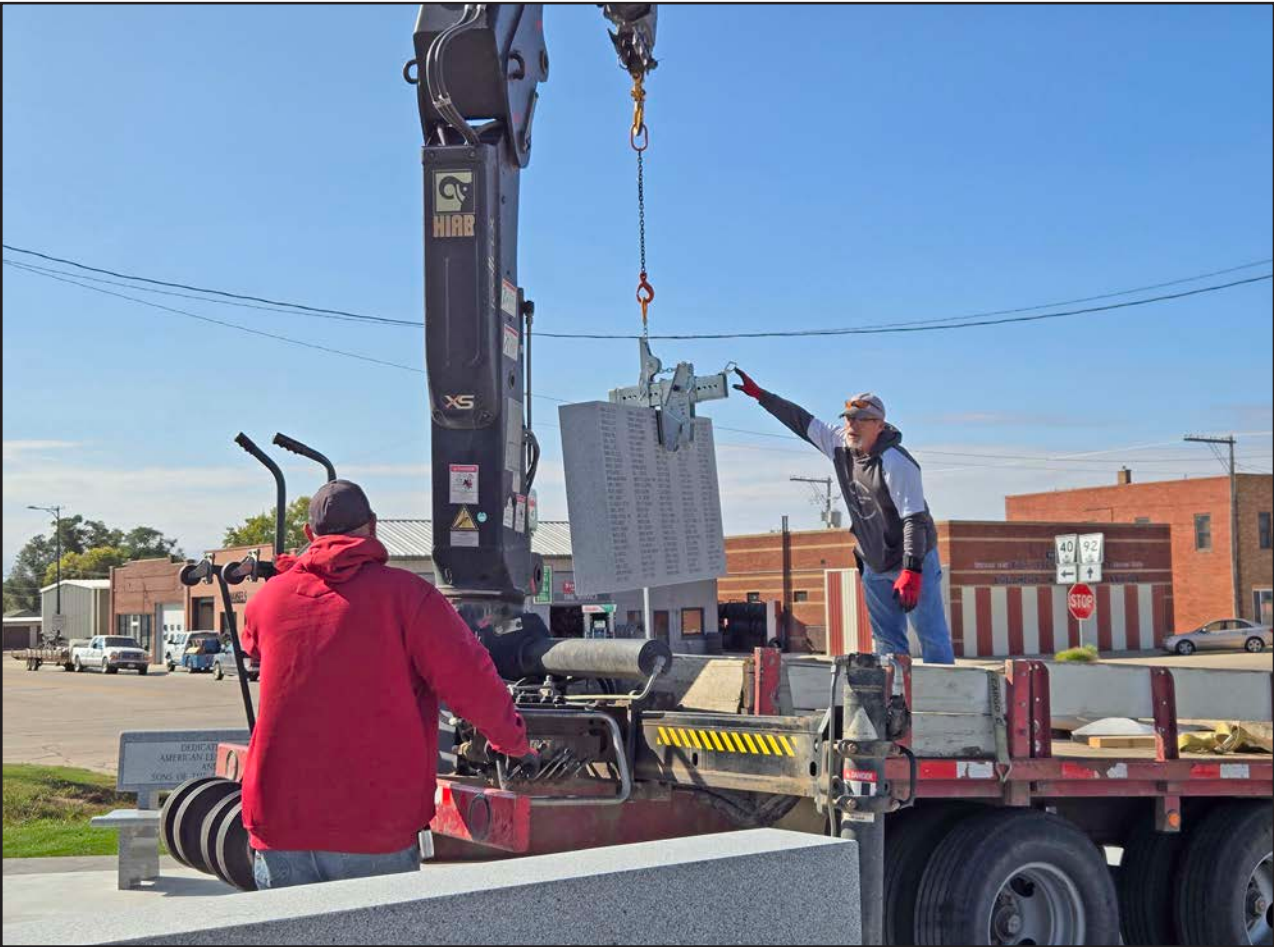
Using a boom truck, Palmer Monument workers lift an almost 5,000 lbs. engraved monument off the truck bed at the site of the Arnold Veterans Memorial. - Debbie Connelly photos
